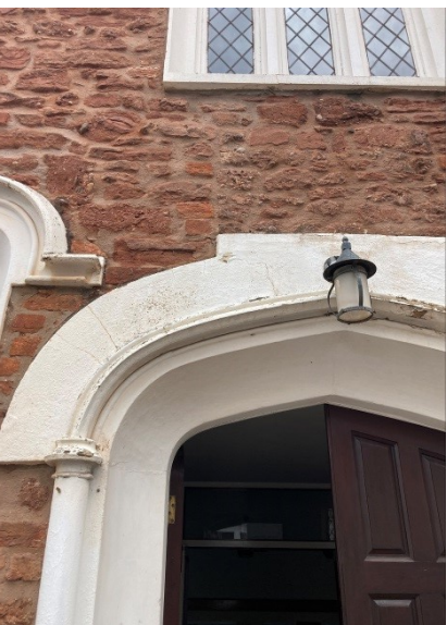
Figs 5 and 6 Minor damage to stone caused by inappropriate paint.
