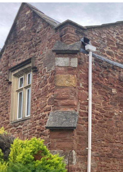
Fig 3 Much of the south wall has cement pointing in various places.
