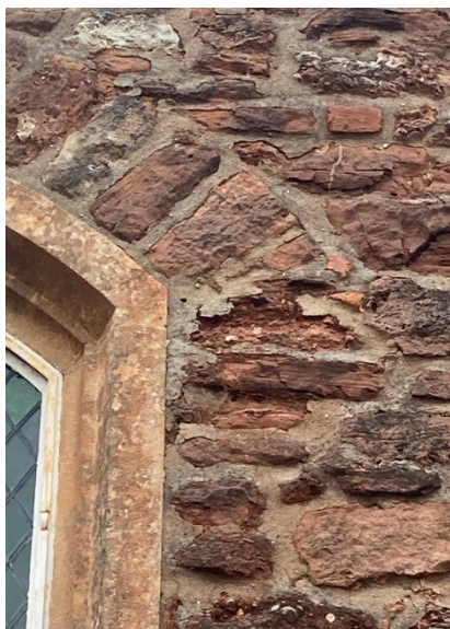
Fig 1 The south wall and south west buttress showing damage to stone from cement pointing.
